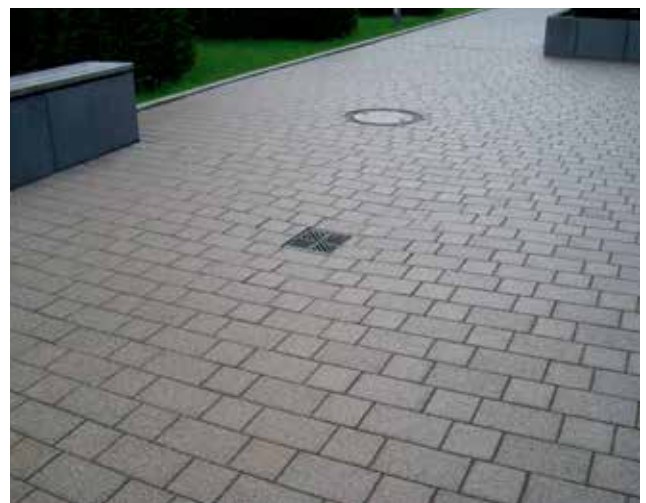
University building in Saarbrücken, Germany
